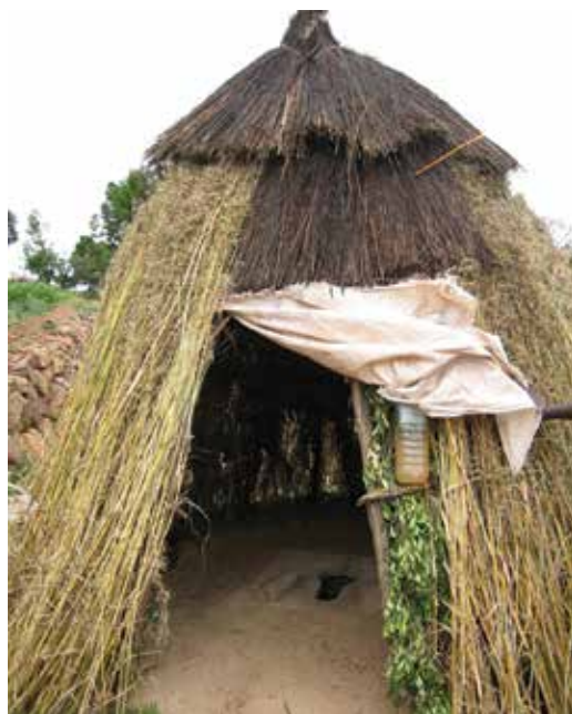
Arborloos are inexpensive toilets that first serve sanitation needs, then later provide a rich source of nutrients for fruit trees. Photo by CRS staff.
